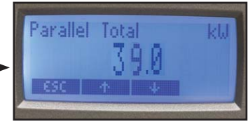
Display full system output from any UPS
