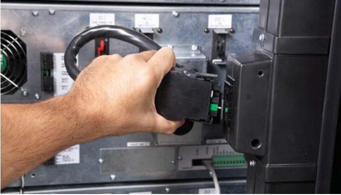
Adding modules is a simple plug-and-power procedure for IT personnel with safety approved connectors.
