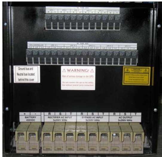
Figure 1: Photo of ac and dc fuses and terminals (50 kVA model)
